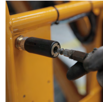
5 Compressed air line
